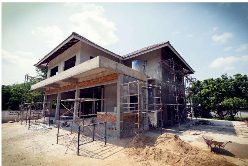
The house is being constructed from a reinforced concrete frame with brick and block masonry infill walls. The house has strip foundations. The upper floor is constructed using reinforced concrete slabs. The roof is pitched and tiled and will include solar panels for both hot water and electricity.
