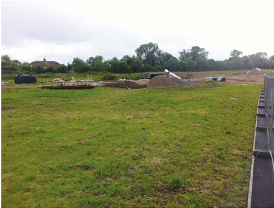
Figure 4: Site ready for excavation – view of the site from the south
