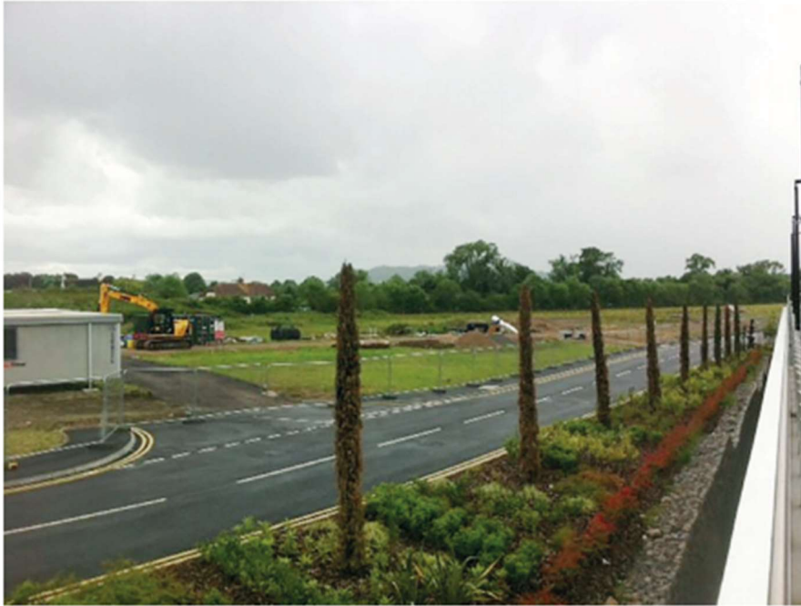
Figure 3: View of the site from the south
