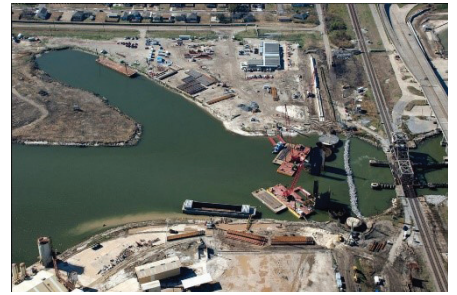
Flood gate (completed in 2012)
