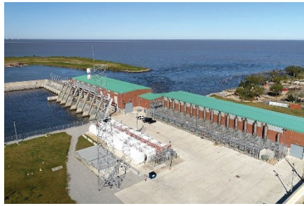
Water pump stations (completed in 2017)
