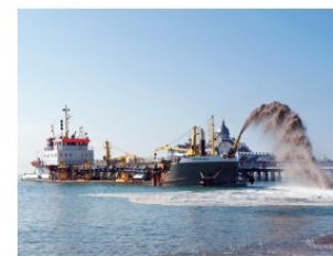
Photo 2 Beach replenishment high maintenance cost and £20 per cubic metre so could be quite expensive.
