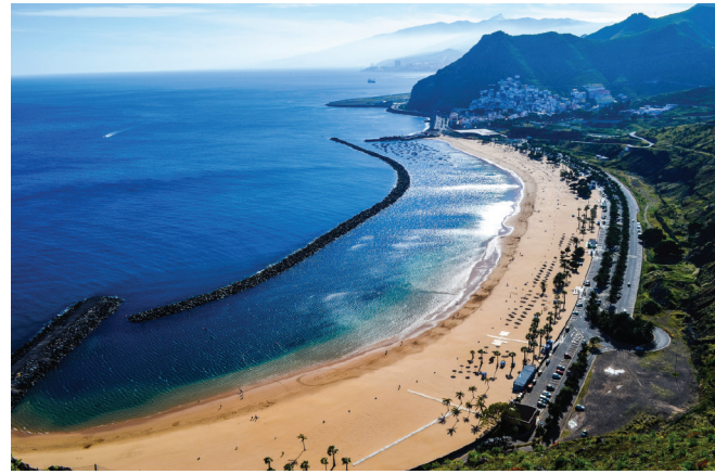
Photo 4. Offshore Breakwater. Medium maintenance cost. High cost per metre, £2,500 – £7,000.
