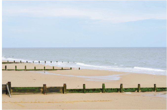
Photo 2 Beach Groynes: Medium maintenance cost. High cost per metre, £1,600 – £4,700.
