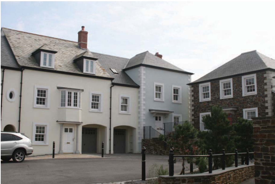
Figure 16 – What new housing in Grampound might look like. This housing was built by Rosemullion Homes 13 km away; it won awards for traditional style and materials e.g. slate
