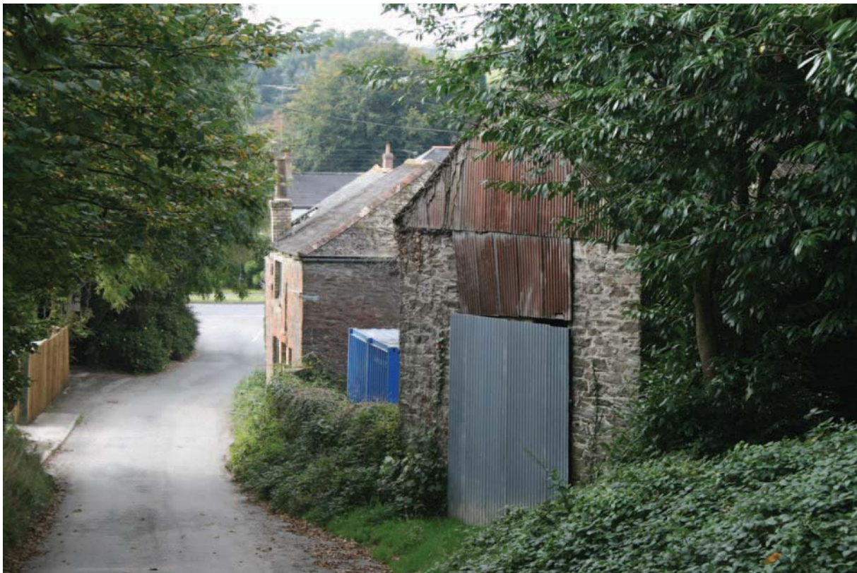
Figure 12 – Some of the buildings occupied by the Pet Supplies store. Several buildings here are unused
