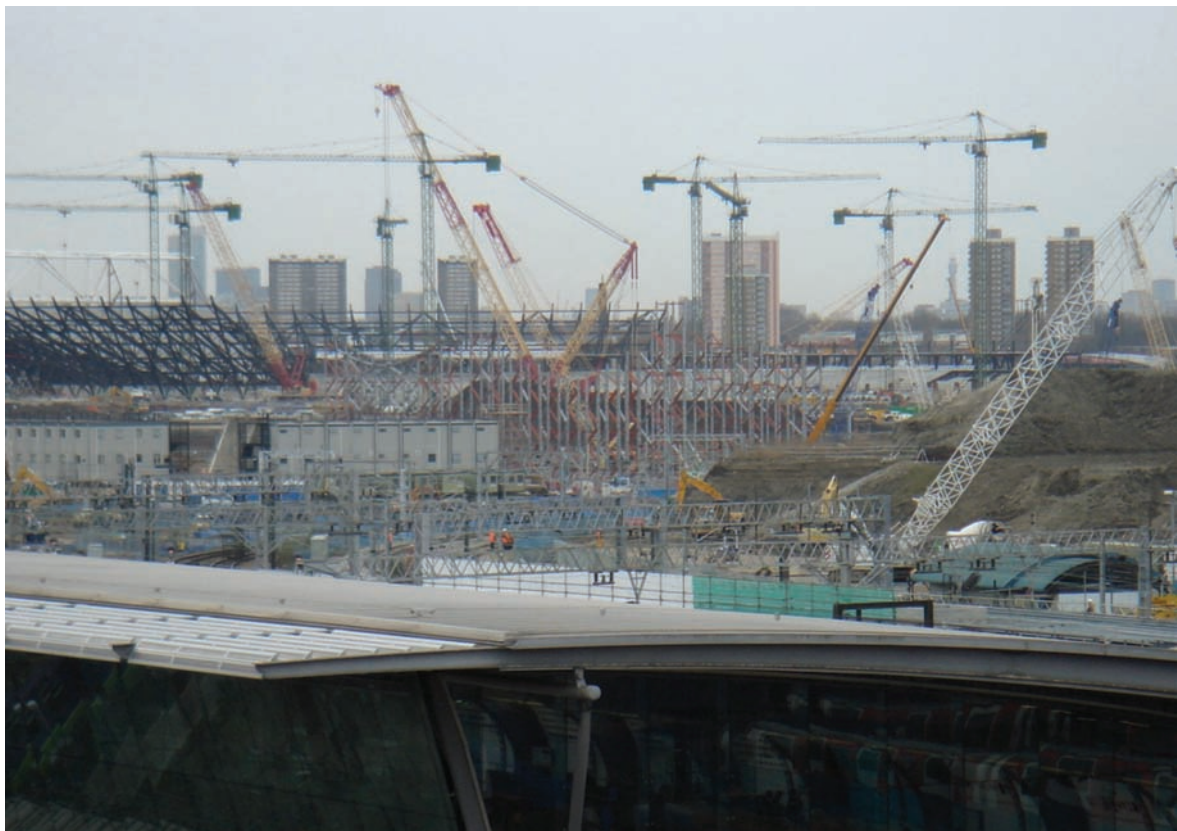
Figure 16 – Building the Olympic Stadium – a boom for construction jobs
