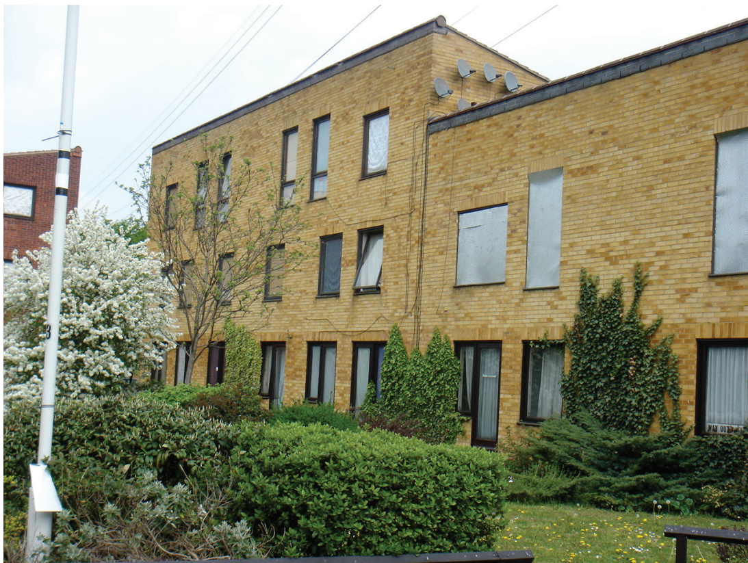
Figure 21 – Clays Lane Community Housing (2007) before clearance. As residents moved out, windows were boarded up
