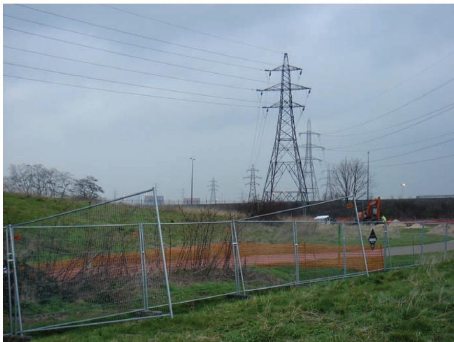
Figure 26 – Electricity pylons before power lines were buried underground
