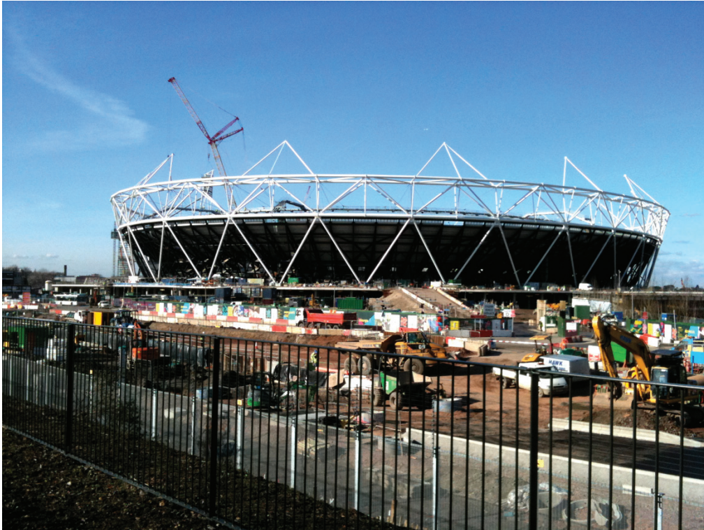
Figure 28 – The Olympic Stadium roof – made out of unwanted gas pipelines
