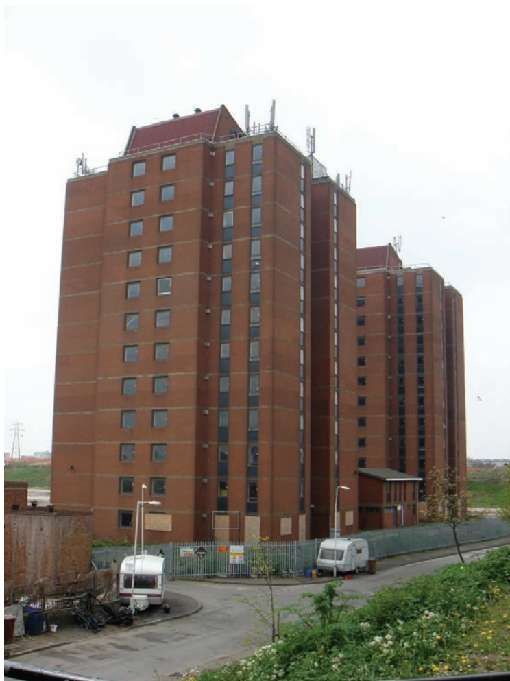
Figure 19 – Student halls of residence in Clays Lane in 2007 before clearance
