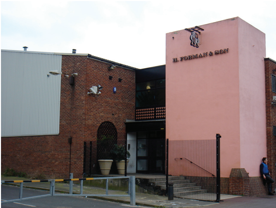
Figure 11 – Forman's smoked salmon factory in 2007, now demolished
