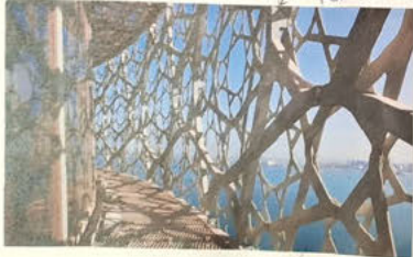
original function of mashrabiya screens = gives protection from heat and sun but allows air through
