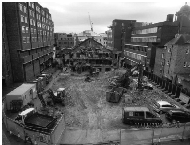
Figure 3: View from south of site during demolition of industrial buildings
