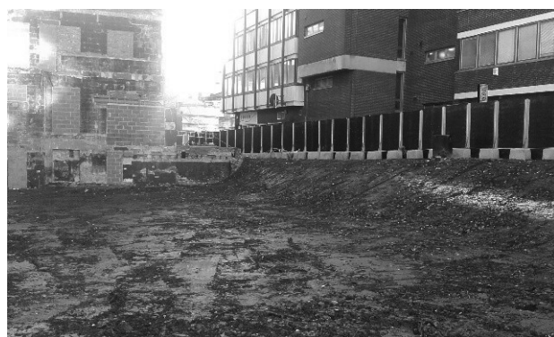
Figure 4: Site excavated to reduced levels – view from south of site
