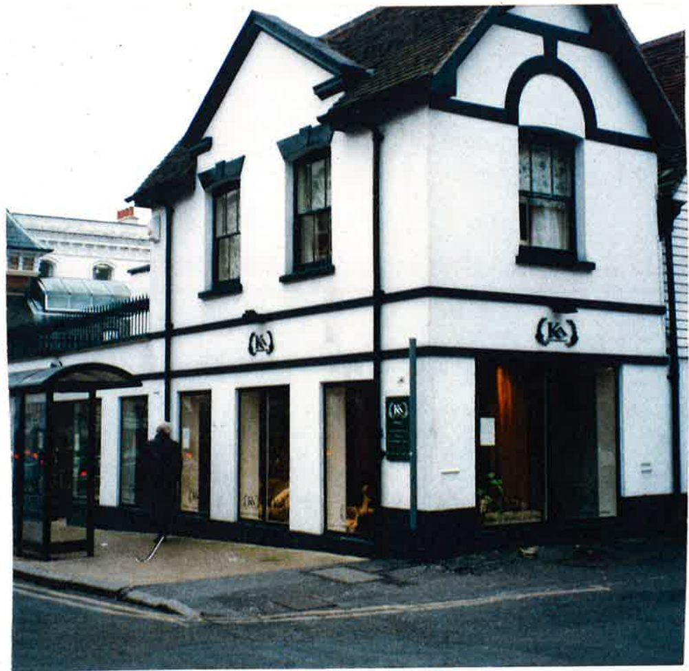
Photo showing the site of the 'Guildford Four' Bombing in the early 1970s, now a Furniture Store, in North Street -
