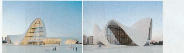
Figure 3 (Heydar Aliyev Centre) & 4 (Heydar Aliyev Centre)
