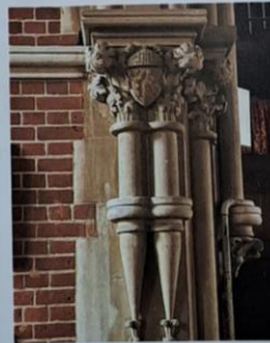
Figure 26: College Chapel column section
