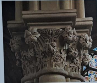
Figure 24: College Chapel Column section
