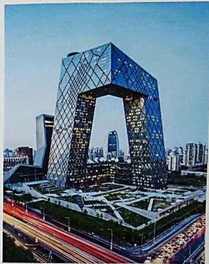
CCTV headquarter - Koolhaas.
